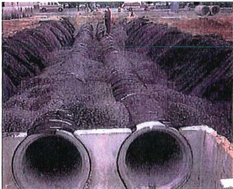
Figure 4 Exfiltration Pipe System (Picture provided by Oldcastle Precast)
