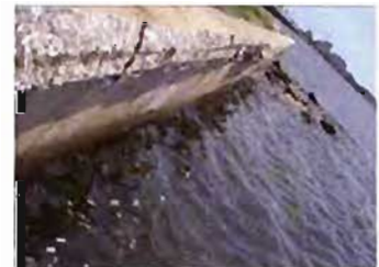
Existing Damaged Seawall
