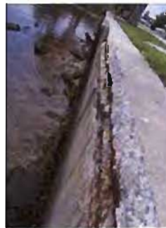
Existing Damaged Seawall
