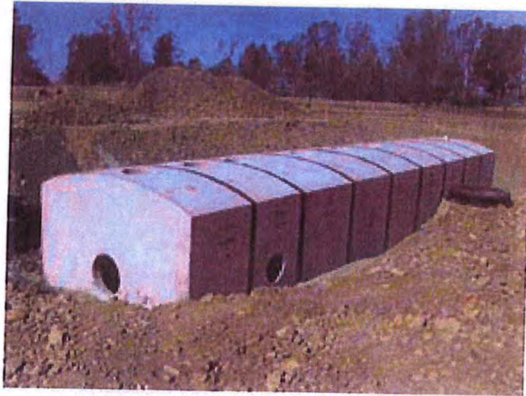
Figure 7 Stormwater Detention Vault System with Effluent Filtration (Sand Filtration)
