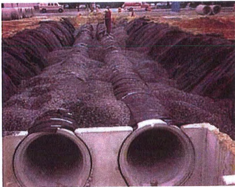
Figure 4 Exfiltration Pipe System (Picture provided by Oldcastle Precast)
