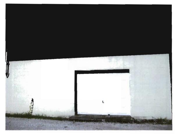
EAST SIDE OF BUILDING - WORK TO BE DONE: REPLACE PANELING, PAINT BUILDING, ADD STUD WALL FRAMING, ADD ARCHITECTURAL ROOF AND ADD ASPHALT PAVING
