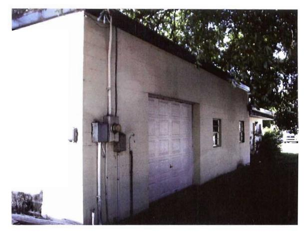
EAST SIDE OF BUILDING - WORK TO BE DONE: REPLACE PANELING, PAINT BUILDING, ADD STUD WALL FRAMING ADD ARCHITECTURAL ROOF
